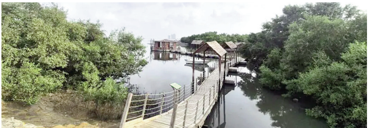
The creek running beneath the Mangrove Biodiversity Park's boardwalk shows visible contamination — dark, sediment-heavy water carrying the combined odour of industrial effluent and raw sewage. The stench reaches you before the view does
